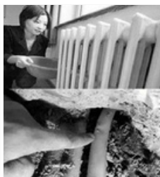
Heating Pipes/ Underfloor Heating Pipe Leaks
