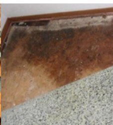
Leak Under The Floor
