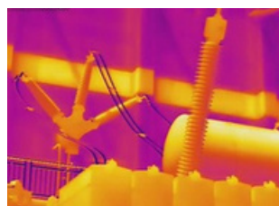
Isolating Switch
